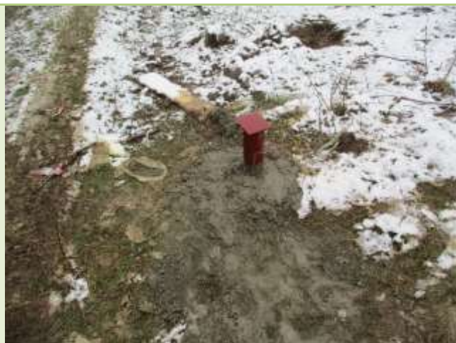
T2-8 BH-1, Piezometer
