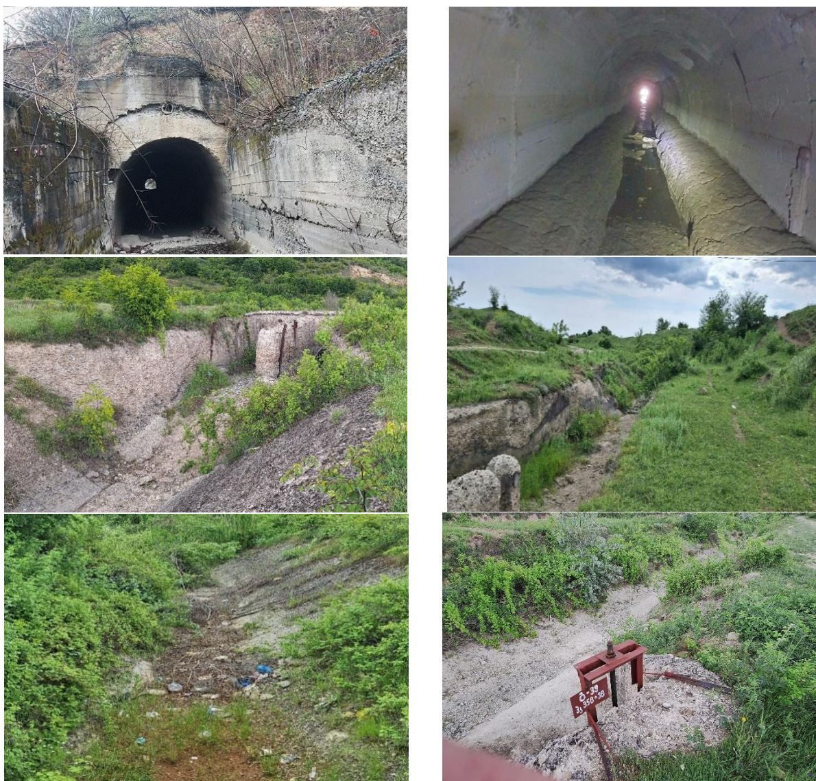
Figure 11. Condition of the Main Canal as of 2025 13
