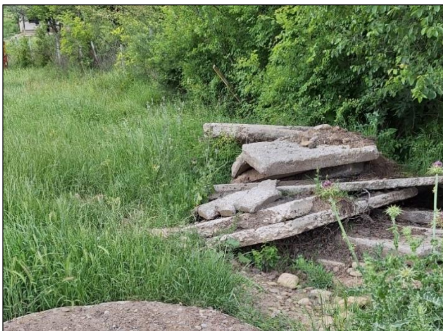
Figure 36. Small Quantities of Concrete Debris Adjacent to the Project Corridor, 2025
