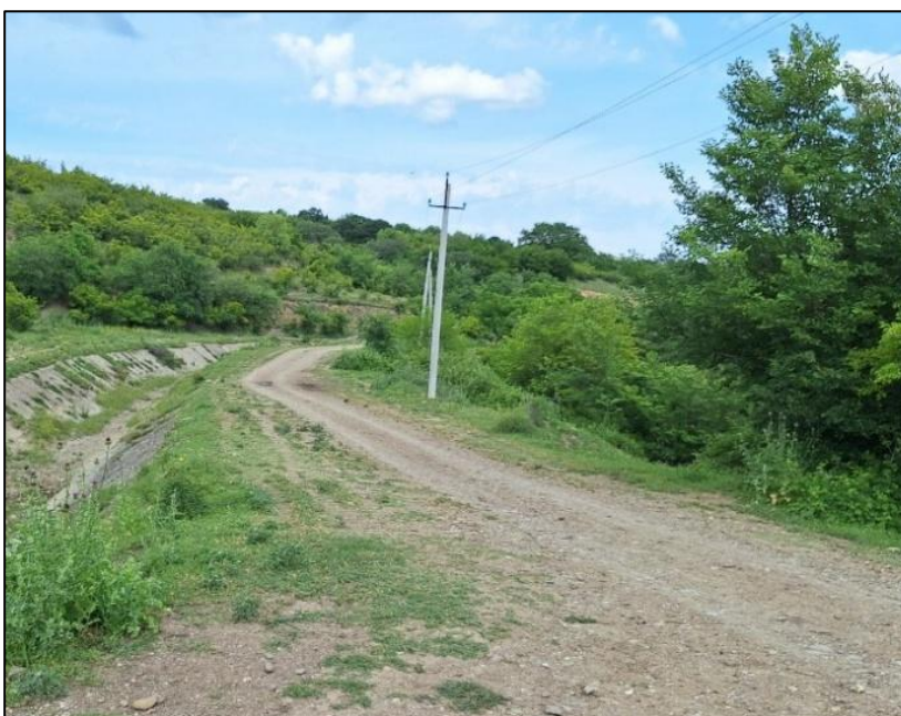
Figure 27. Low Voltage Power Lines Located near the Main Canal
