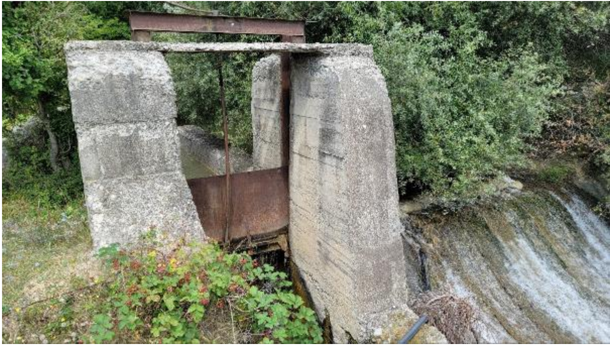
Existing Hydraulic structures
